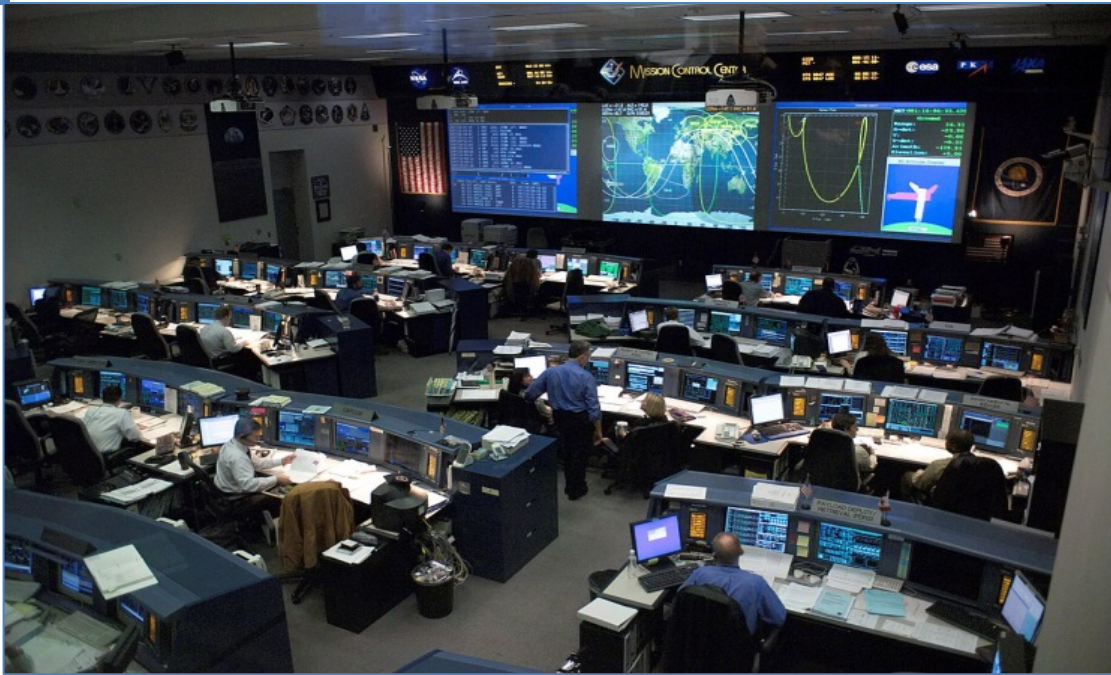
Figure 2.8: example control room
