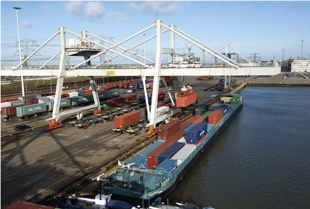
Figure 7.54: Barge feeder crane at ECT Delta terminal (source: ECT)
