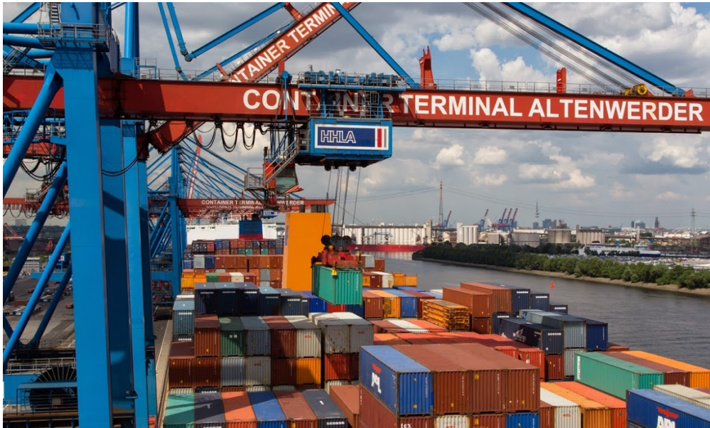
Figure 7.20: Post Panamax STS crane at Container terminal Altenwerder
