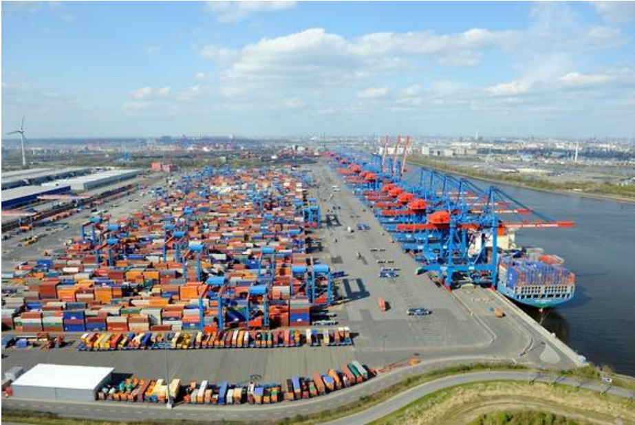
Figure 7.42: Overview of the container terminal Altenwerder (source: CTA)
