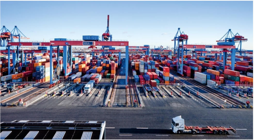
Figure 7.32: Rail Mounted Gantry (RMG) in stack of Container Terminal Altenwerder (Hamburg, Germany) (source: hhla.de)
